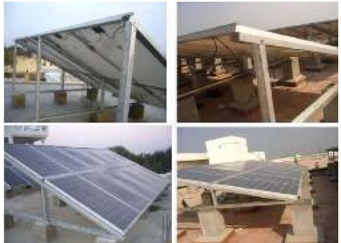
Figure 4.7: GI mounting structure
