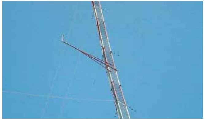
Figure 20: Installation Arrangement of Sensors at Keti-Bandar Mast
