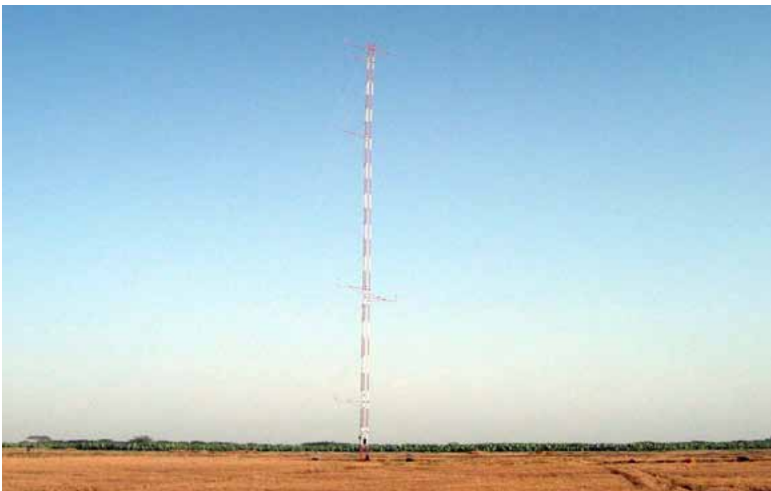
Figure 19: AEDB-UNDP (WEP) Keti-Bandar Mast.
